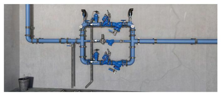
Pressure Reducing Station, featuring BERMAD BC-70F-P Strainers to protect each branch from foreign debris, a redundant, parallel branch to minimize the possibility of total water shut-off and a low flow bypass branch for low demand operation. For information on the other BERMAD products in this system please see the product data sheet for the BERMAD BC-720-P and BERMAD BC-73Q-P.
