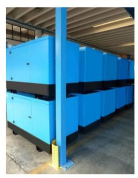
Soundproof and weatherproof canopy, made with structural steel, thickness between 1,5 and 4,5mm. Painted with epoxy dust RAL5015.
